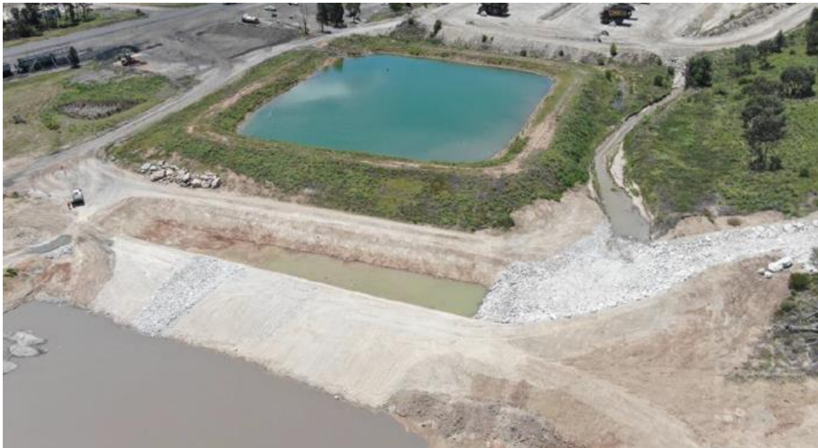
Figure 5 SB16A Forebay constructed and inlets rock lined
